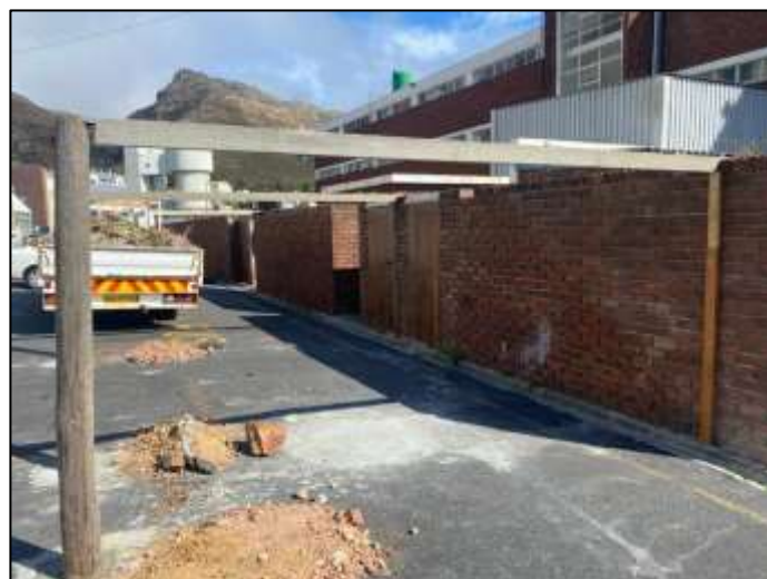
Figure 11. Construction has started on a large secure area where galley waste bins can be stored at West Yard.
